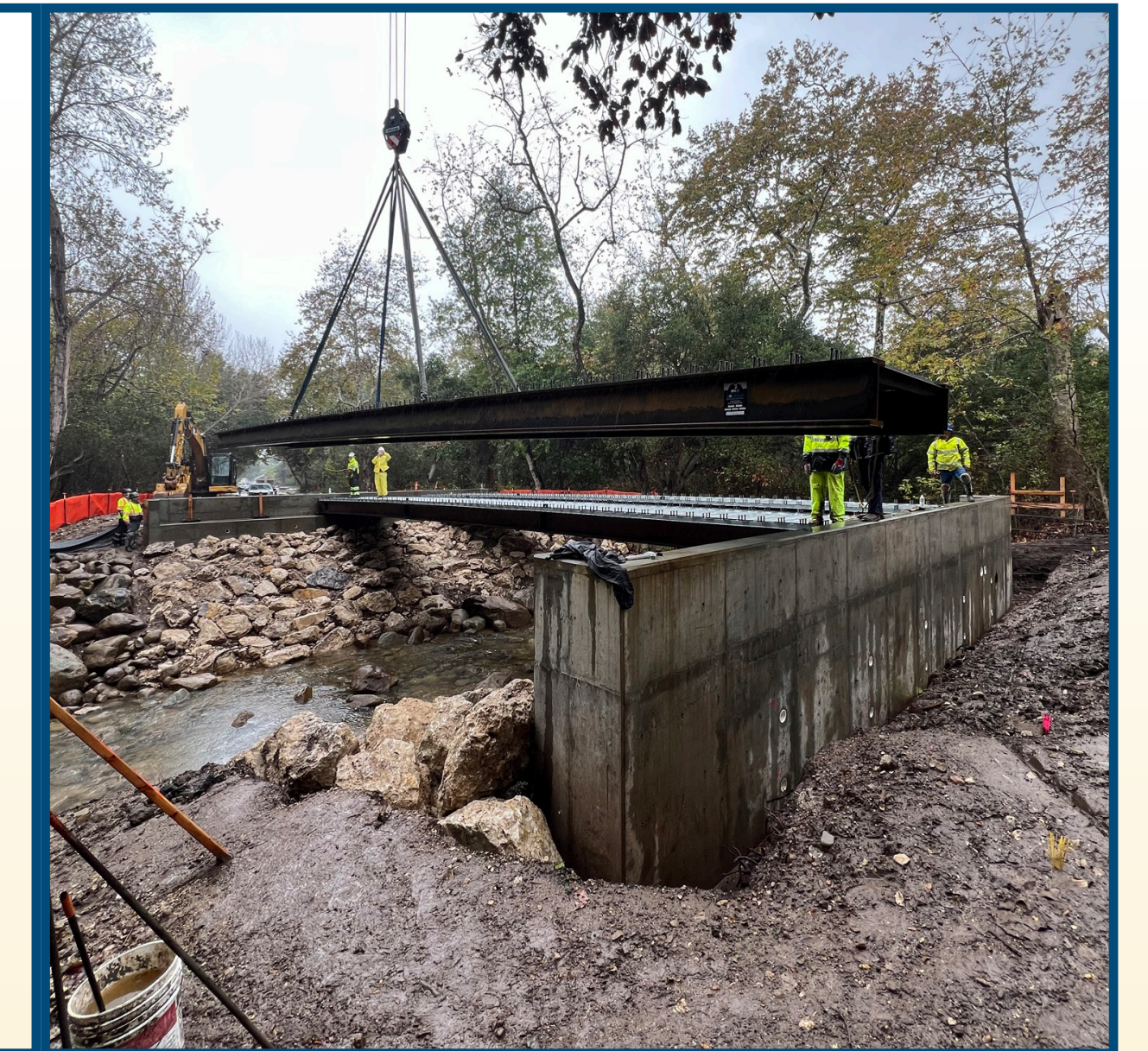
El Capitán entrance bridge construction. Photo source: Parks, January 2026.
